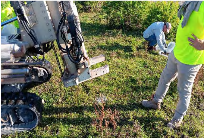
Photo 5: MW-4 DPT install begins
