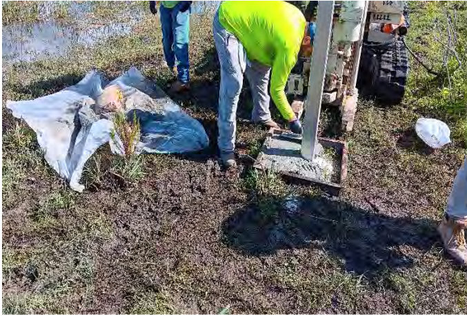
Photo 9: MW-3 riser and concrete pad install.
