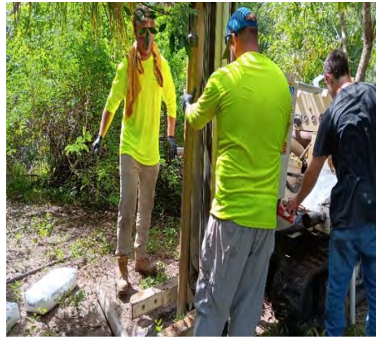
Photo 12: MW-2 DPT install.
