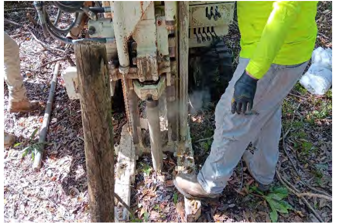
Photo 10: MW-1 DPT install
