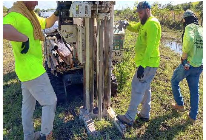
Photo 8: MW-3 DPT install
