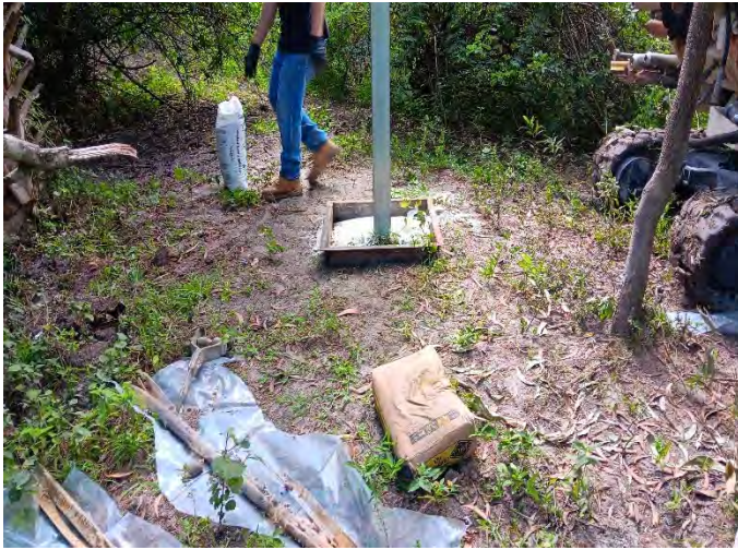
Photo 13: MW-2 riser and concrete pad install.
