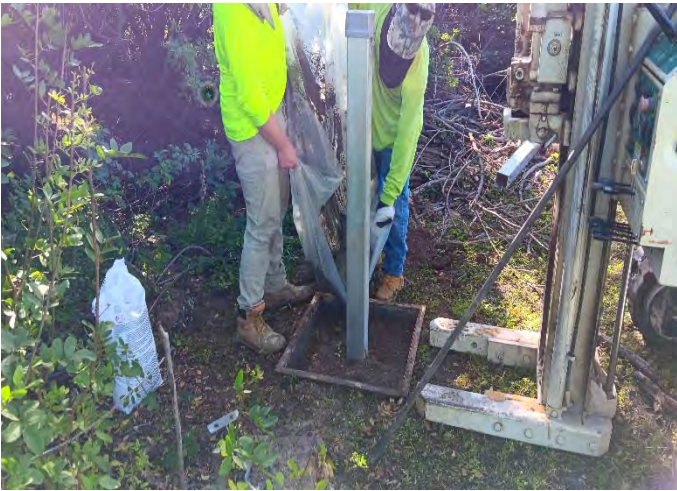
Photo 7: MW-6 concrete pad and riser install.
