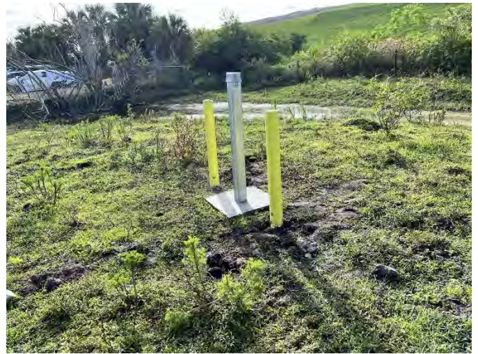
Photo 22: Final view of ballads around MW-4
