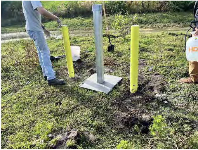
Photo 21: Ballard install around MW-4
