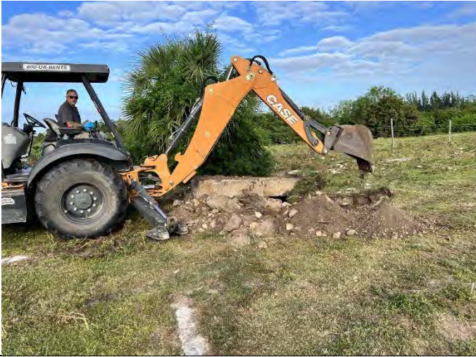
Photo 17: Test Pit (TP) #1
