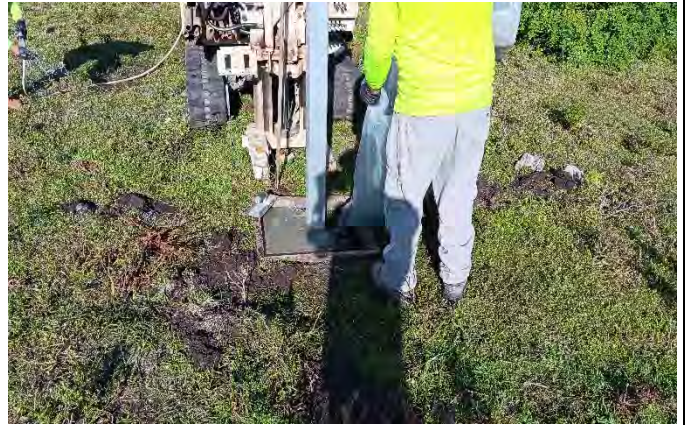
Photo 6: MW-4 riser and concrete pad install.
