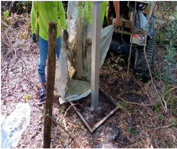
Photo 11: MW-1 riser and concrete pad install.
