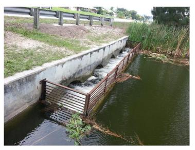
Figure 23. High flows through Weir 20 on 7/16/2014. Culverts are almost full after a short rainfall event. High-water marks are visible well above the culvert crests.
