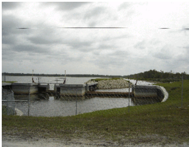
Storm water detention pond and discharge control structures for the new terminal at Southwest International Airport.
