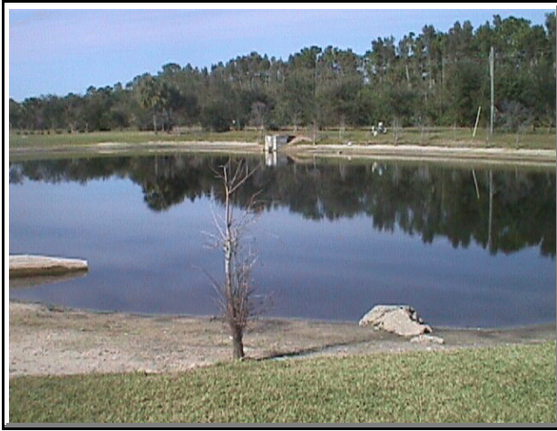
A detention pond in a residential subdivision. Note the control structure in the background.
